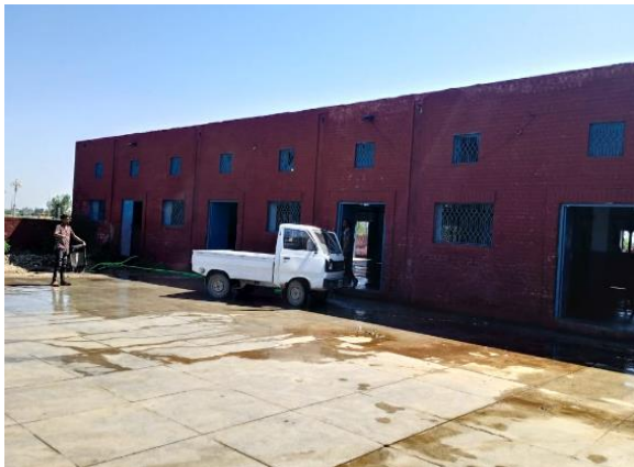
Figure 22: Front View of the Slaughterhouse
